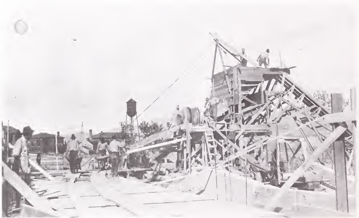
Jefferson County funded the construction of a new two-span reinforced concrete T-beam bridge in the fall of 1917. The bridge was located on Montana Highway 69 on the southern outskirts of Boulder. This photograph shows the concrete mixing plant. The Boulder School and Hospital is located in the background (Montana Historical Society).
